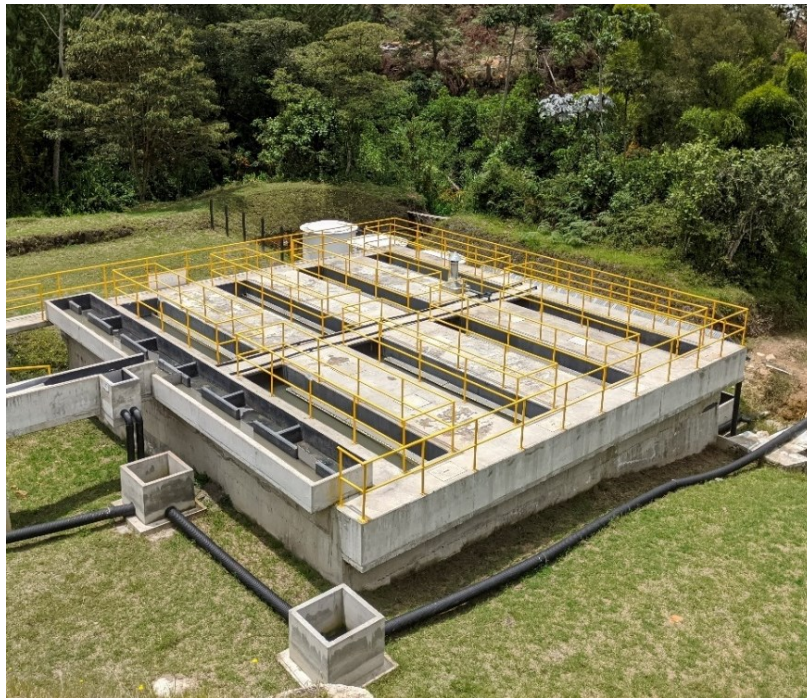
Fig 39. Reactor UASB.
