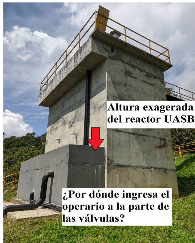
Fig 45. Reactor UASB
